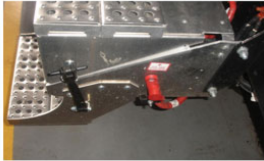
Step that contains batteries with red jump post
