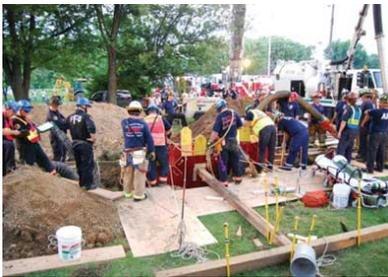
(4) The buttress system as part of the shoring plan.
